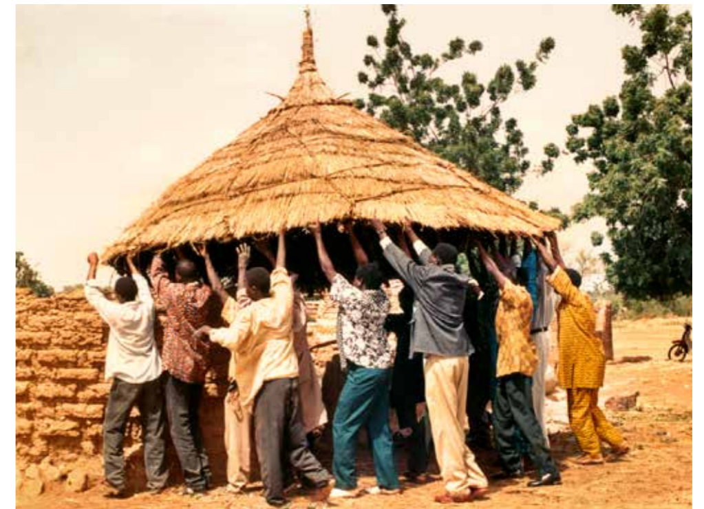
Palhé ' helping to fix a roof. Guibaré, Burkina Faso, 2004.
